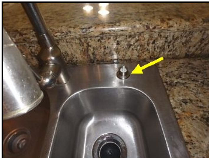
soap dispenser missing handle
