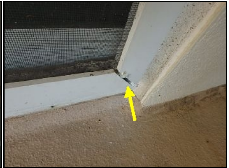
Bottom corners are starting to sepearate
