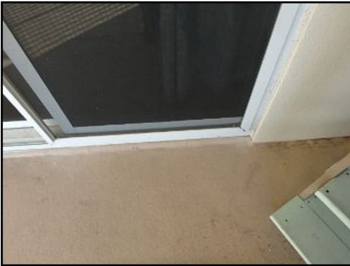
Bottom corners are starting to sepearate
