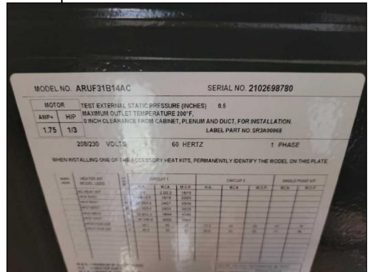
No defects noted at the time of inspection
