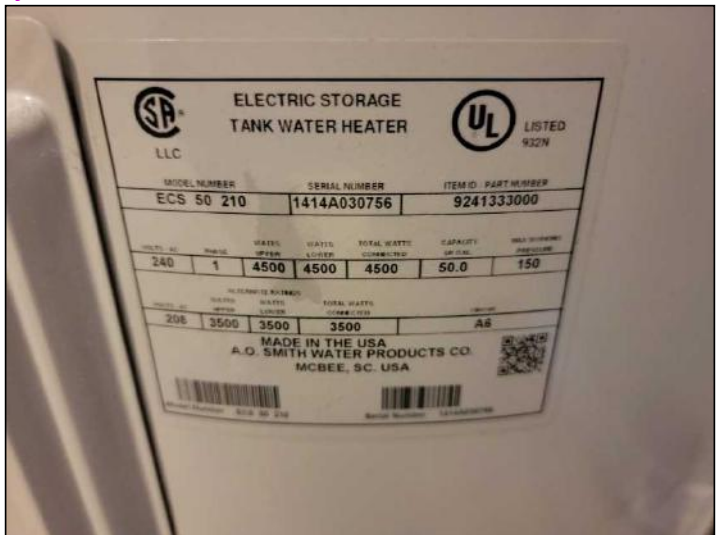
Tank is in satisfactory condition -- no concerns.
