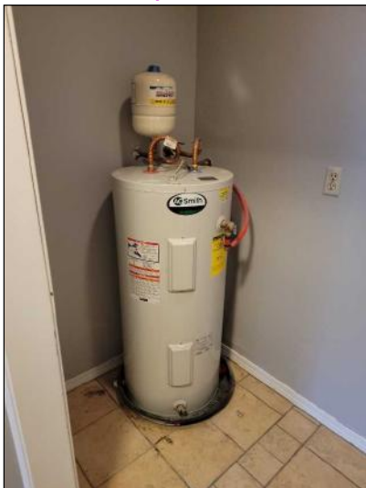
Tank is in satisfactory condition -- no concerns.
