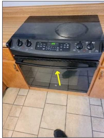
Oven door handle loose. Repair
