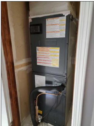
No defects noted at the time of inspection
