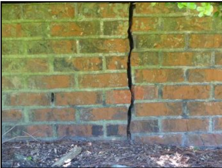
Large cracks were observed at the visible foundation walls. Repairs can be expensive and further settling or damage could occur. Recommend a Structural Engineer to provide a detailed analysis before the close of escrow on the structure.
