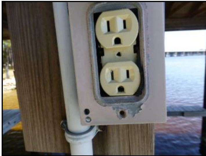
outlet on boat dock does not have a weatherproof seal.
