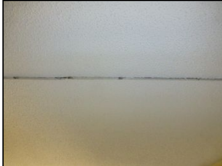
Living room ceiling has separated at the drywall seam. Have repaired as necessary.
