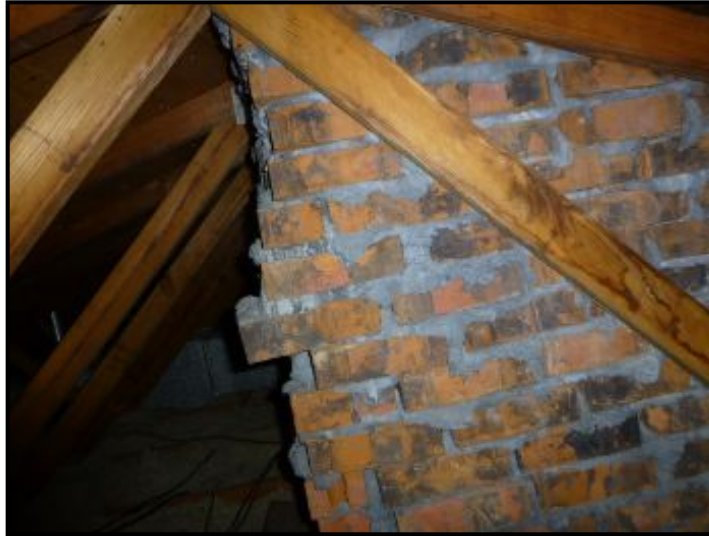
Brick and mortar deterioration observed; repair advised.
